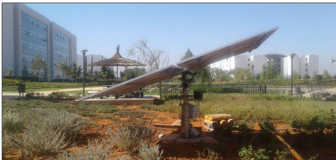
**1,2 kW Pilot project off-grid solarwater pumping irrigation systems – Rabat - Morocco**
